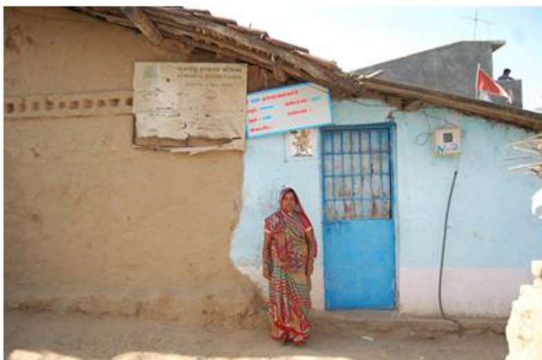
Work in progress: Navliben's pucca-kachha dwelling
