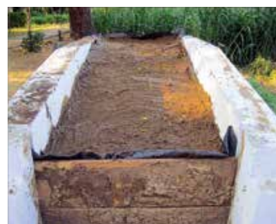
Fully sealed silo pit
