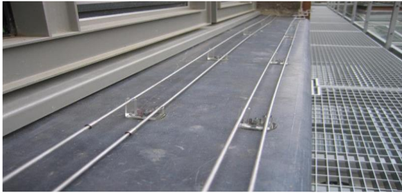
Electric bird deterrent system learns the birds over time to stay away from the protected areas
